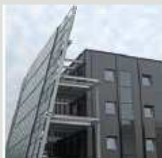
Retrofitted multi-family house Kapfenberg (AT)
